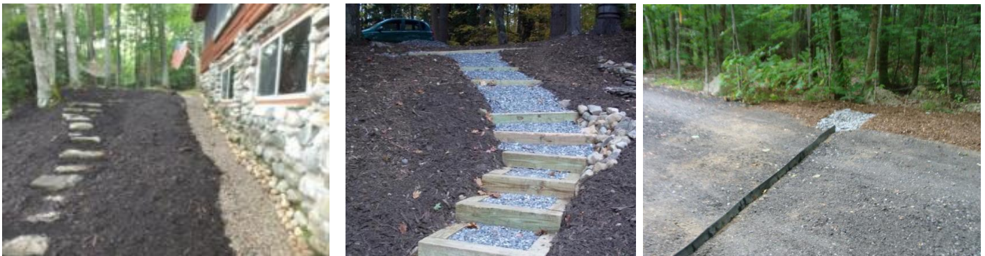
Examples of conservation practices for residential properties and driveways: 1) Erosion control mulch and roof dripline trench, 2) Erosion control mulch and infiltration steps, 3) Rubber razor. (Photos: AWWA, J. Jespersen)
